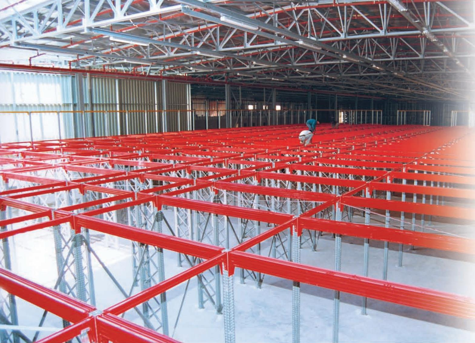
■ The Super 6 upright has eight connection points along four faces, allowing the interconnection of this element in all four directions.
